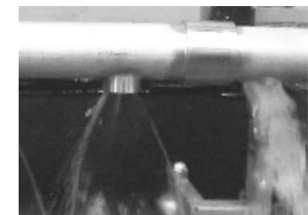
Foreign objects inside the pipe are flushed out through the drain.
